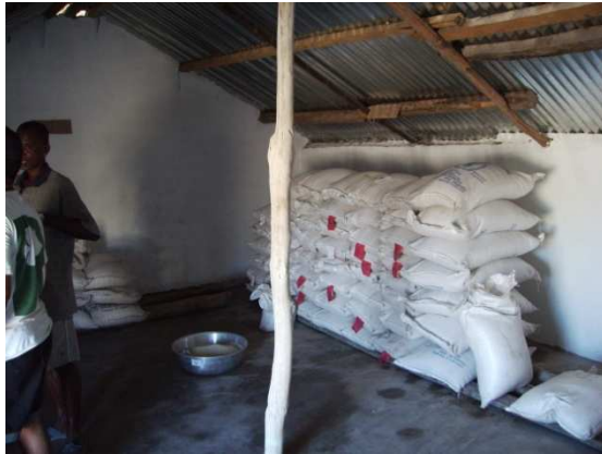
Repaired storeroom - now cement floor
