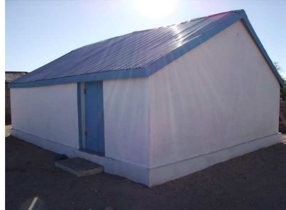
Repaired food storeroom
